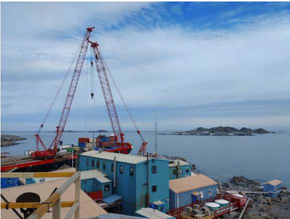
Pier Construction in January, 2022. Image Credit: Marissa Goerke
